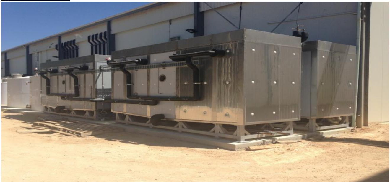
Figure.11 PCM Tanks
