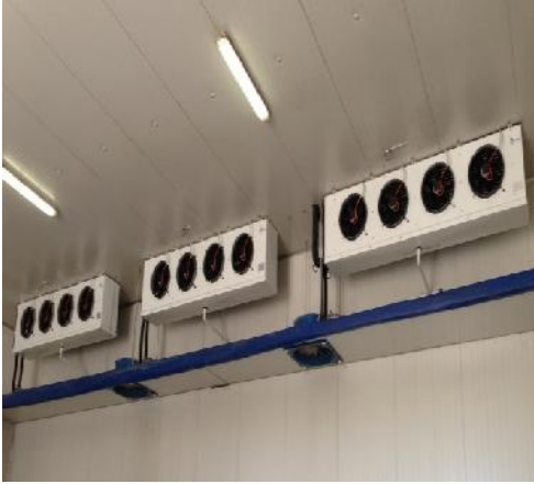
Figure.12 Quikcool Evaporators
