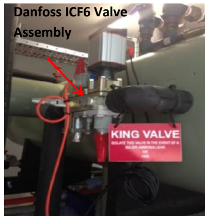
Figure.6 ICF 6 Make up valve
